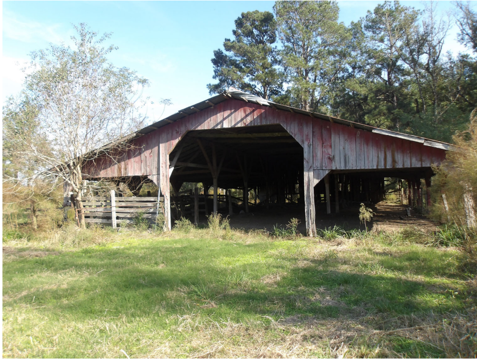
Photo 17: PL11 of agricultural structure facing east taken 11/26/2024
