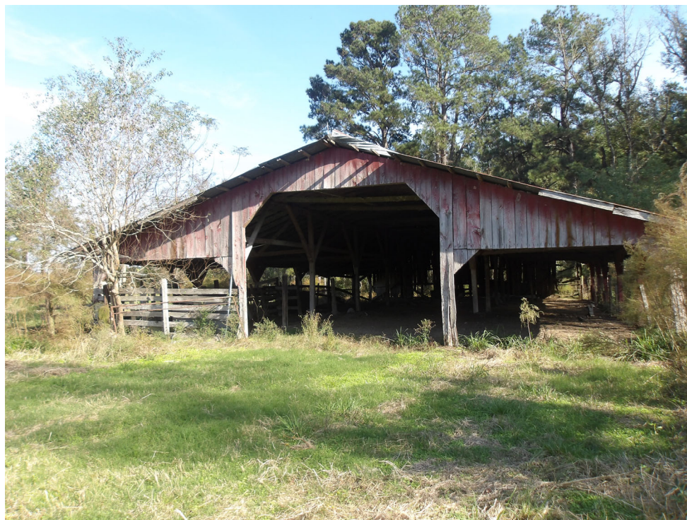
Photo 17: PL11 of agricultural structure facing east taken 11/26/2024
