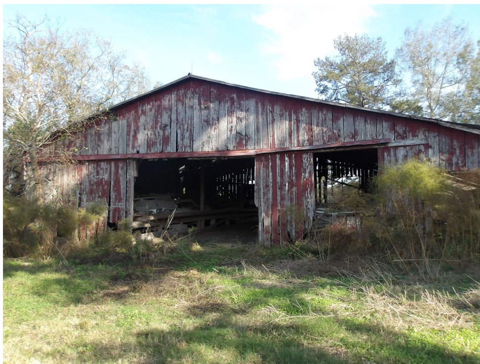
Photo 20: PL14 of agricultural structure facing east taken 11/26/2024
