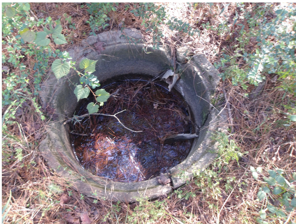
Photo 14: PL9 of in-ground structure facing south taken 11/26/2024
