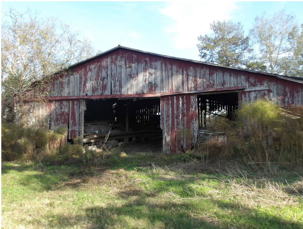
Photo 20: PL14 of agricultural structure facing east taken 11/26/2024
