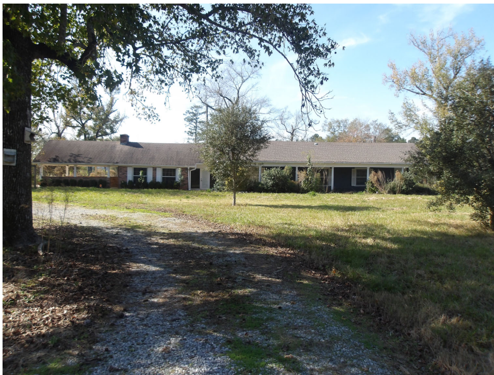
Photo 11: PL7 of homesite facing west taken 11/26/2024
