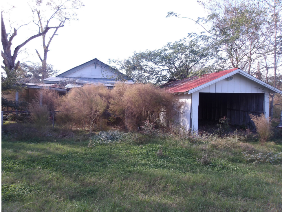
Photo 21: PL15 of homesite facing west taken 11/26/2024
